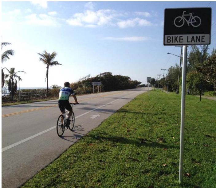
Bicyclist using a bike lane with an R3-17 sign (Credit: Kimley-Horn and Associates, Inc.)
