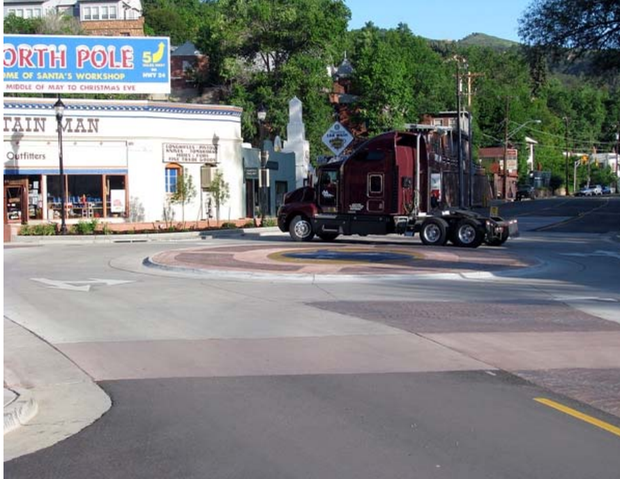
Mini-roundabout (Credit: Ian Lockwood)
