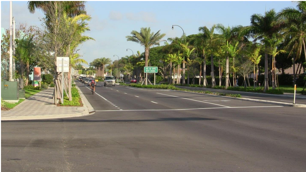
Boulevard example: Hillsboro Boulevard (Credit: City of Deerfield Beach Planning Department)
