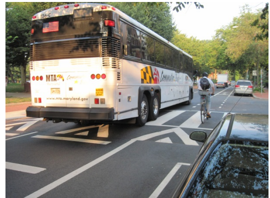
Raised crosswalk (Credit: Toole Design Group)
