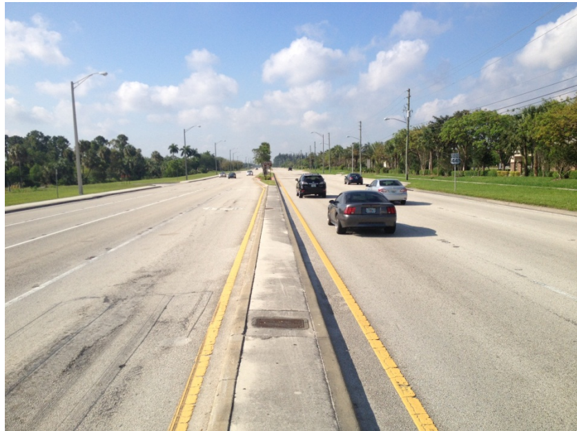
Wide, uninviting boulevard; a typical existing condition (Credit: Kimley-Horn and Associates, Inc.)
