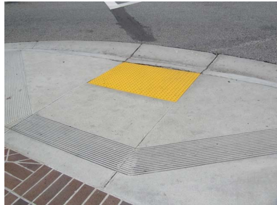
Required truncated domes (Credit: Ryan Snyder)
