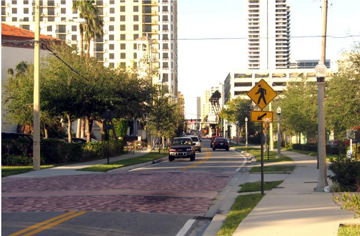
Raised crosswalk (Credit: Ian Lockwood)
