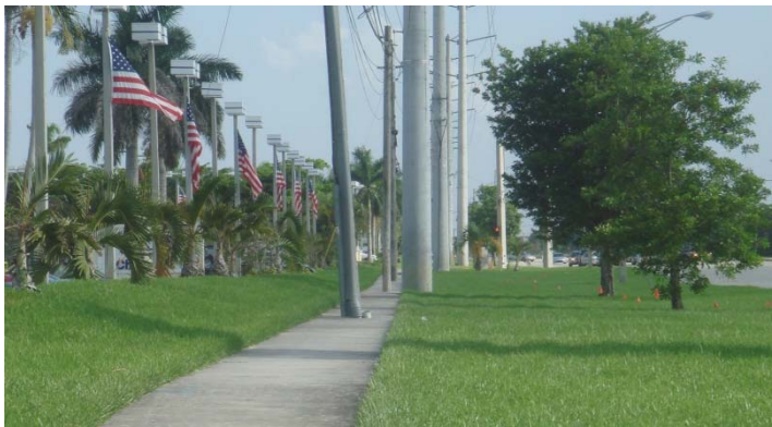
Sidewalks constructed without adequate design guidelines (Credit: Kimley-Horn and Associates, Inc.)
