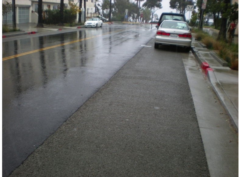
Permeable pavement after a rain event (Credit: Neil Shapiro)
