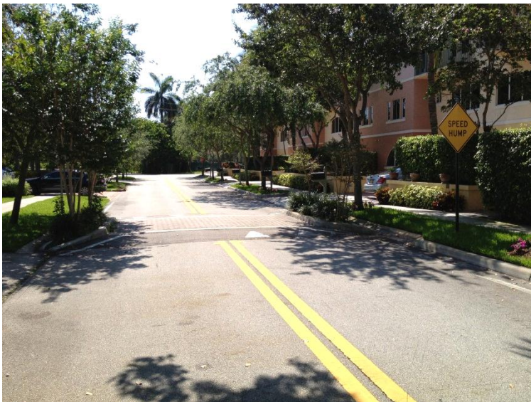
Speed table and lane narrowing with warning sign (Credit: Kimley-Horn and Associates, Inc.)
