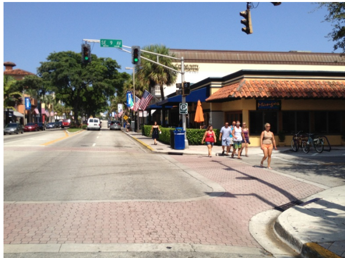
Crossings should be designated on every leg of all intersections in an urban context (Credit: Kimley-Horn and Associates, Inc.)
