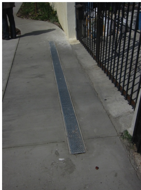
Trench drain in hardscape (Credit: Stephanie Landregan)
