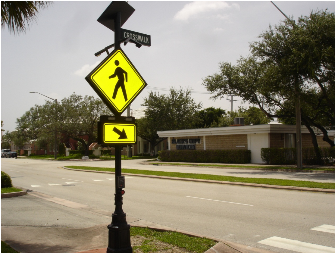
Pedestrian warning sign (W11-2) at a high emphasis crosswalk. Note the yield bars (series of isosceles triangles painted on the approach to the crosswalk).
