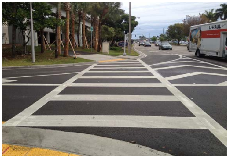
FDOT special emphasis crosswalk; note this design may have been improved by a channelization island for refuge (Credit: Kimley-Horn and Associates, Inc.)
