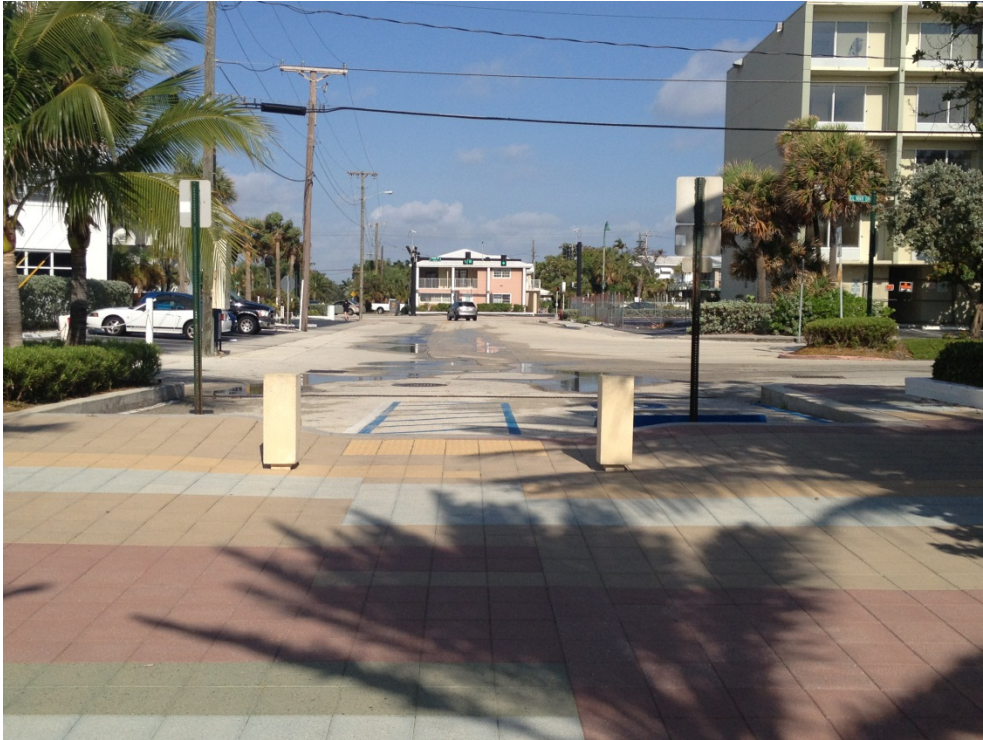
Bollards separate a street-end from the sidewalk (Credit: Kimley-Horn and Associates, Inc.)
