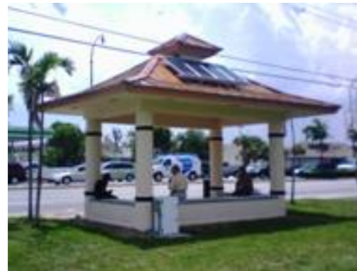
Transit shelter with solar power (Credit: Maribel Feliciano)
