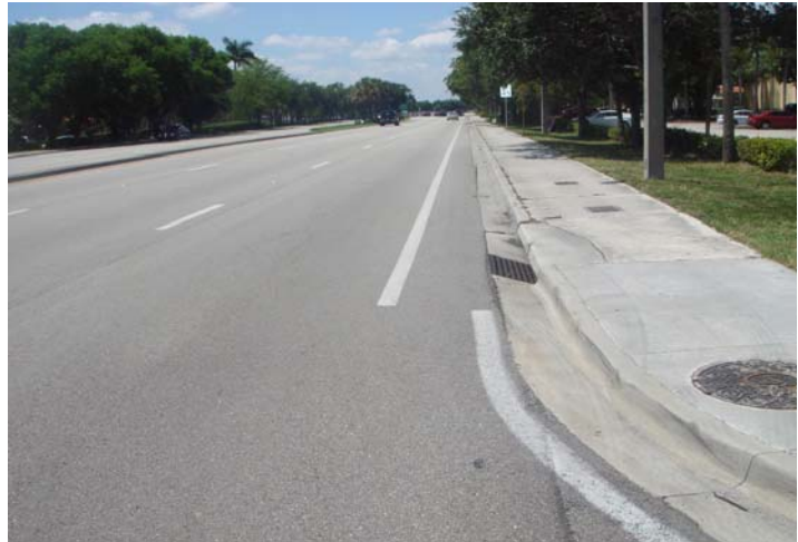
Undesignated lane. Note the corner radius striping, which allows bicycles to enter the undesignated lane.
