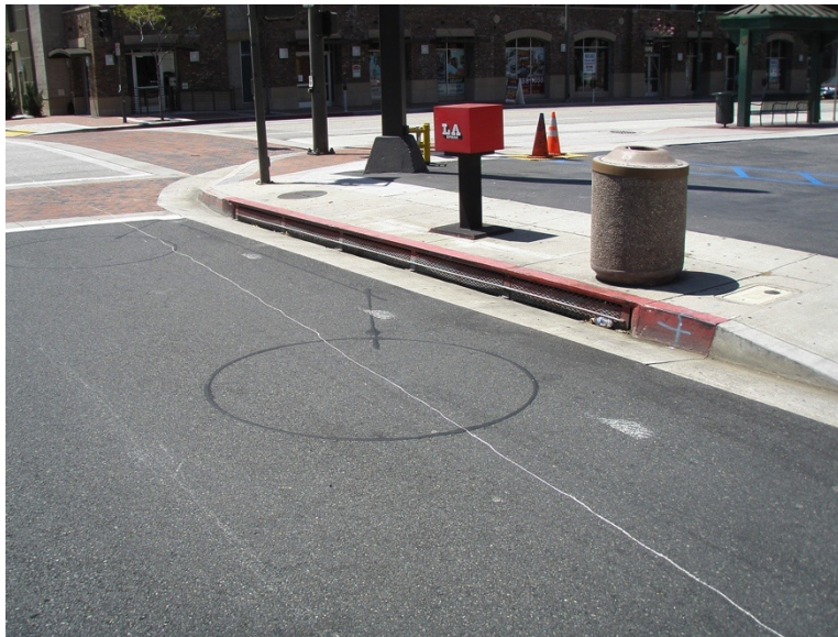
Curb inlet grate catching debris (Credit: Andre Haghverdian)
