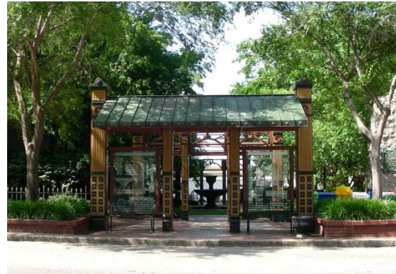
Bus stops should be integrated with their surroundings (Credit: Kimley-Horn and Associates, Inc.)
