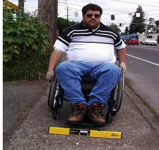
Steep cross slopes create difficulties for wheelchair users. (Credit: Michael Ronkin)
