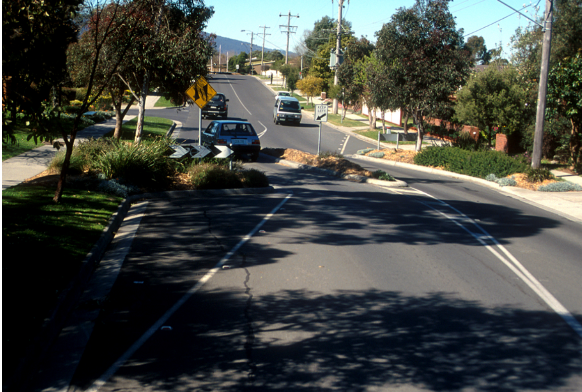
Two-lane chicane (Credit: Michael Wallwork)
