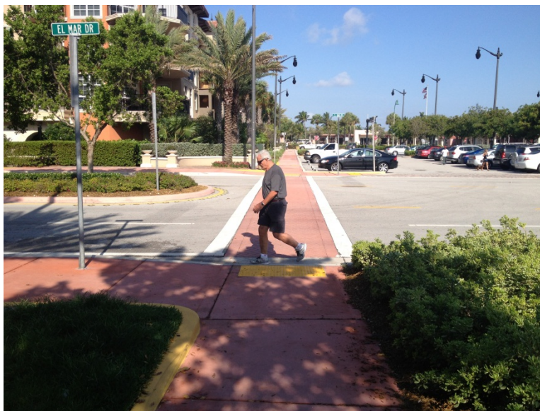
Marked crosswalk. If decorative treatment is applied it shall be bordered by solid white line crosswalk markings. (Credit: Kimley-Horn and Associates, Inc.)
