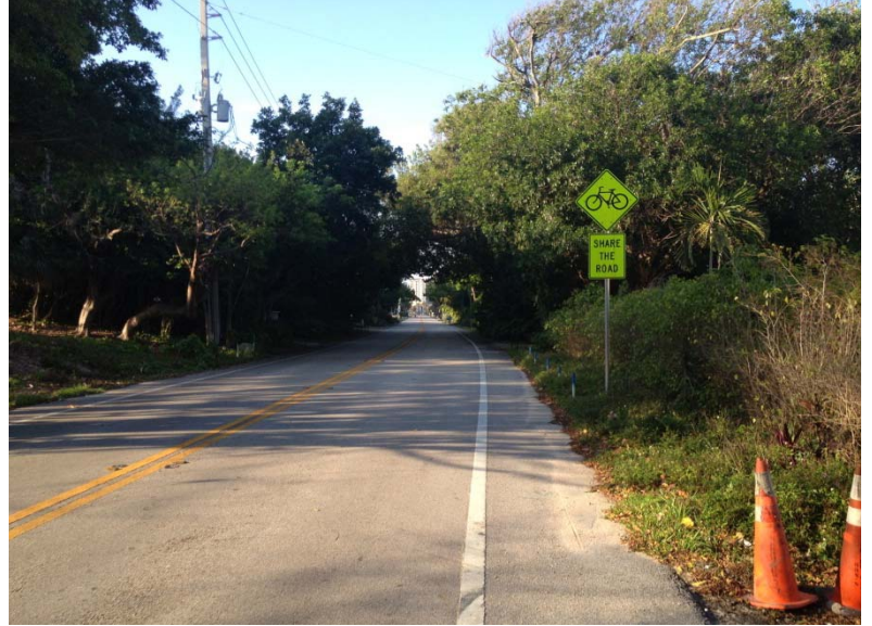
Paved shoulder with Share-the-Road sign assembly (Credit: Kimley-Horn and Associates, Inc.)
