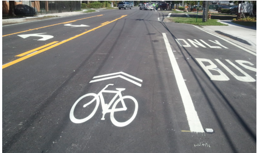
Sharrow pavement marking (Credit: Kimley-Horn and Associates, Inc.)
