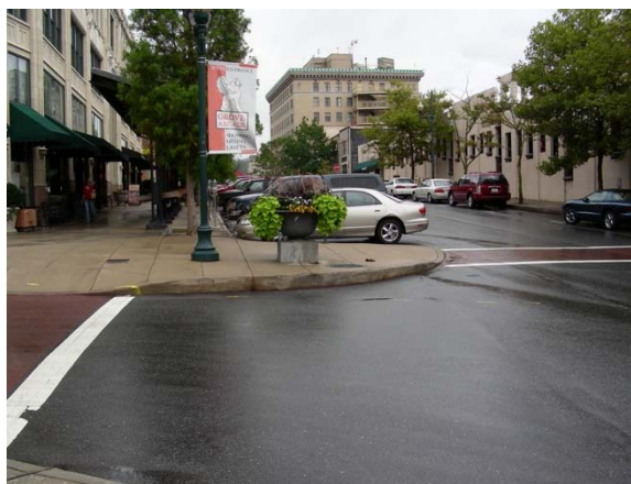
Curb extensions enhance retail districts: Asheville, North Carolina (Credit: Ryan Snyder)
