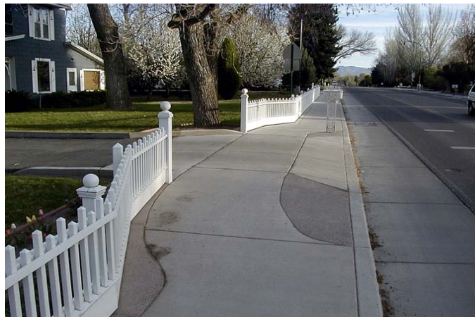
Routing sidewalks around driveway ramps maintains a flush surface. (Credit: Dan Burden)
