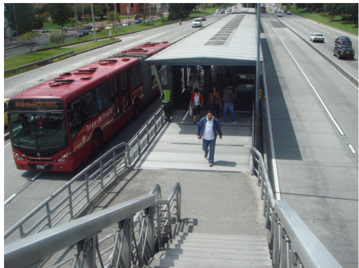
Busway in median with center platform stations: TransMilenio BRT, Bogotá, Colombia (Credit: Stewart Robertson)
